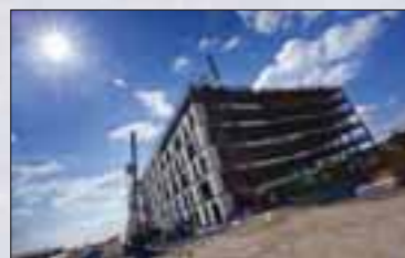
2009 Work began at the new Headquarters for GMP located at Newton Heath, Manchester.
