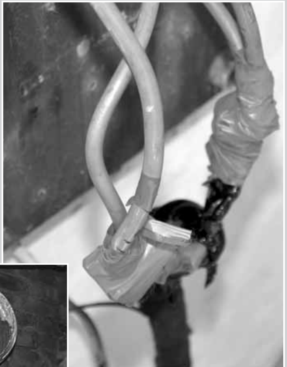
Special venting (left) and unstable wiring (above)
