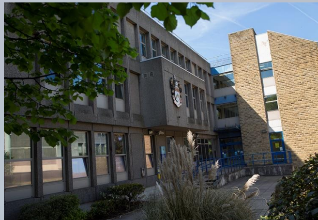
Oldham Police Station, Barn Street
